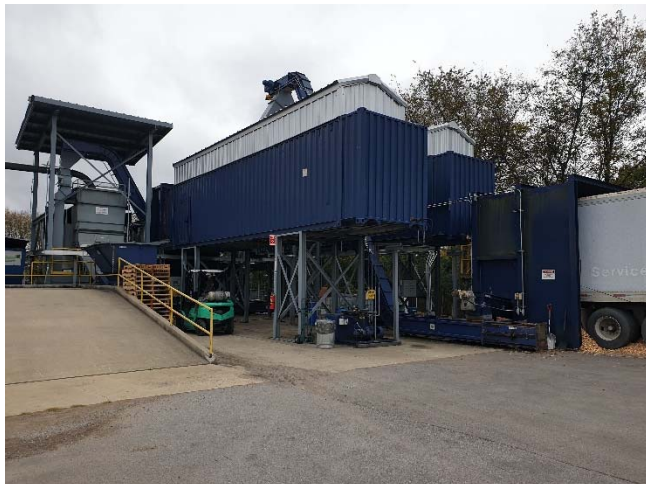
Biomass feed system – TN
