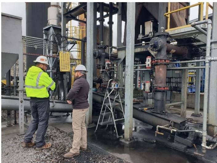
Bottom part of the Gasifier – TN
